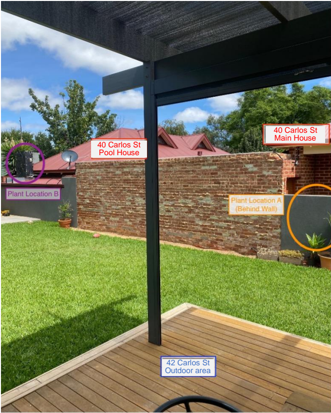
Figure 3 – View of Mechanical Plant locations, from complainant property.
